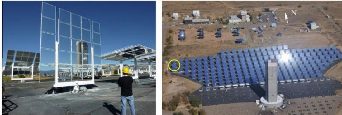
Fig. 1. Left: heliostat 12W14 at the NSTTF in Albuquerque, NM, which was retrofitted with 3M™ Solar Mirror Film 1100. Right: NSTTF heliostat field with location of 12W14 heliostat circled.
